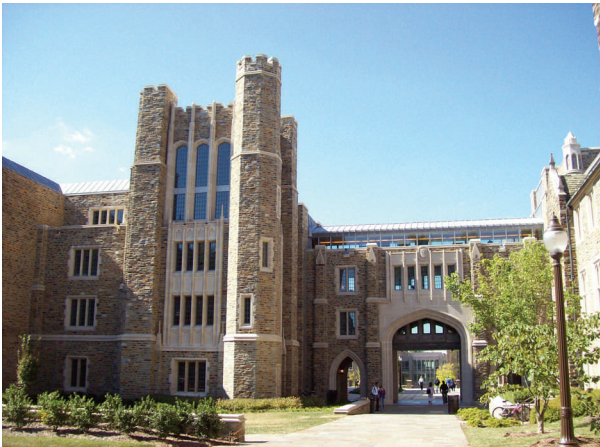
Duke University Perkins Library Renovations and Additions Durham, NC
